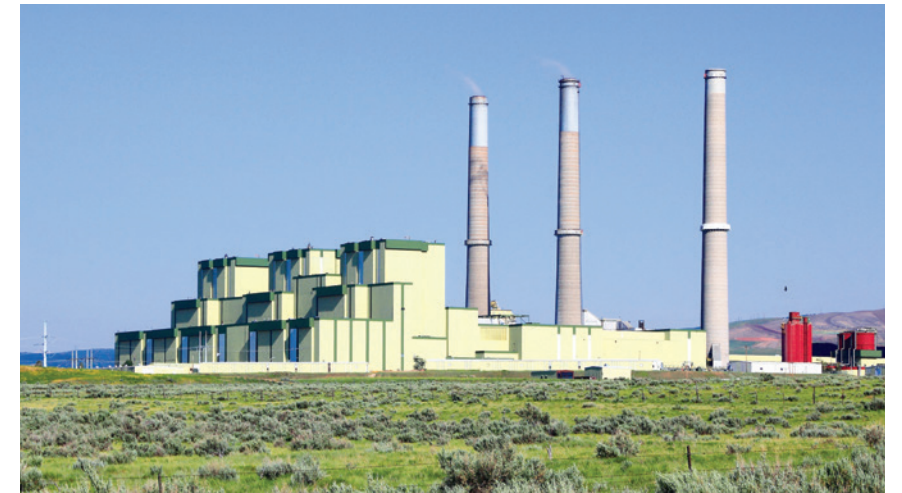
The Craig Station power plant in Moffat County.
